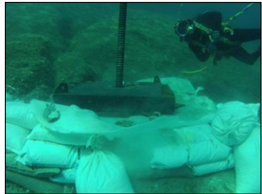
Figure 6 – Diver Installed Grout Bags
