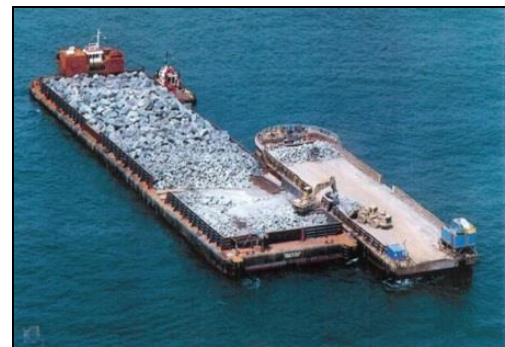
Figure 2 – Side Dump Vessel with Engineered Rock
