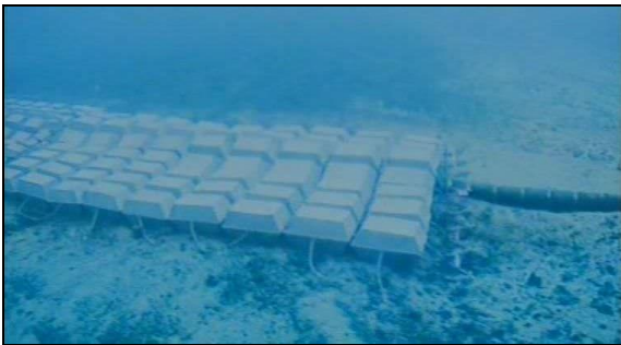
Figure 5 – Concrete Mattress over a Pipeline
